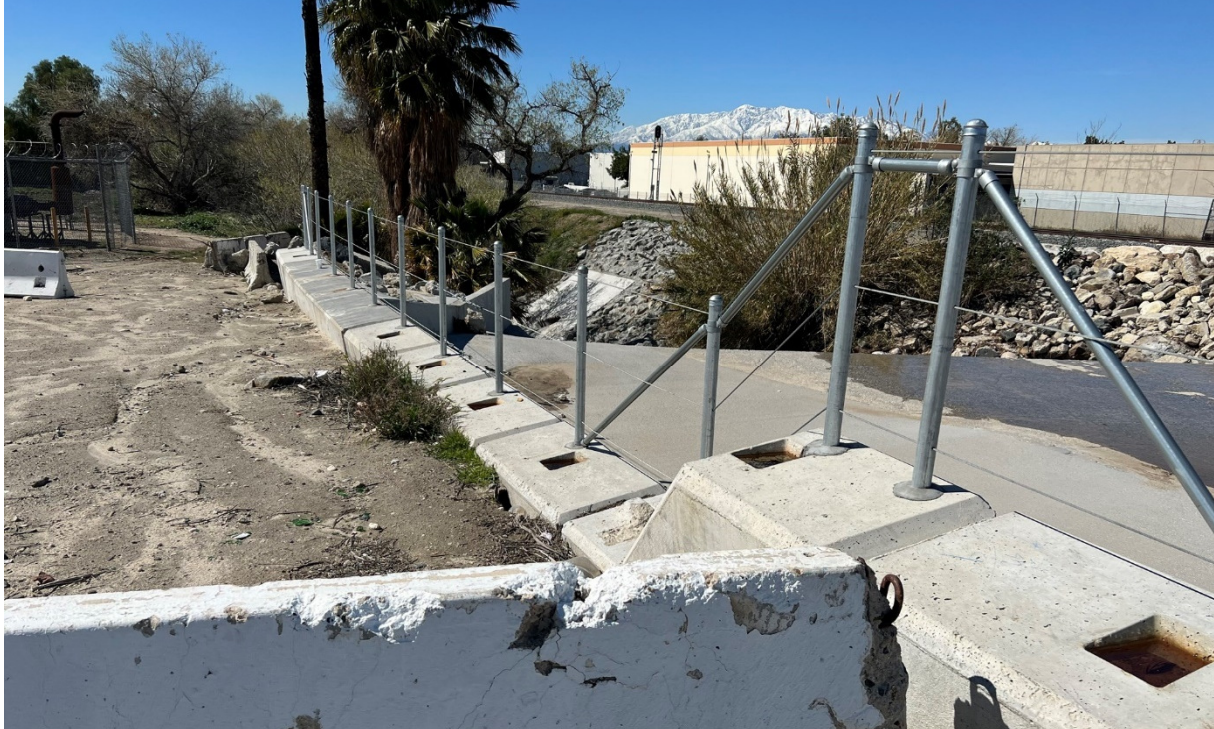
Closer view of drainage channel, northwest of the northern property.
