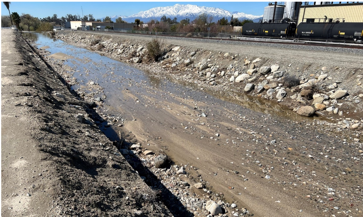
Closer view of adjacent water channel to the north of the northern property.
